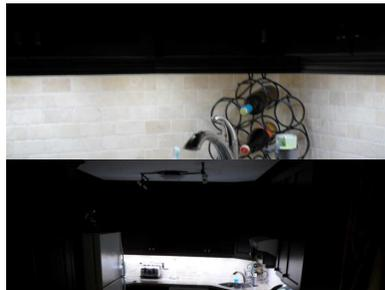
To illuminate the top of her counter, Ms. Doucet has chosen to install the power supply under the counter behind the sink and hide the wire in the wall between the cabinets and countertop. The LED modules are simply fixed under the cabinets beside the light valance.
